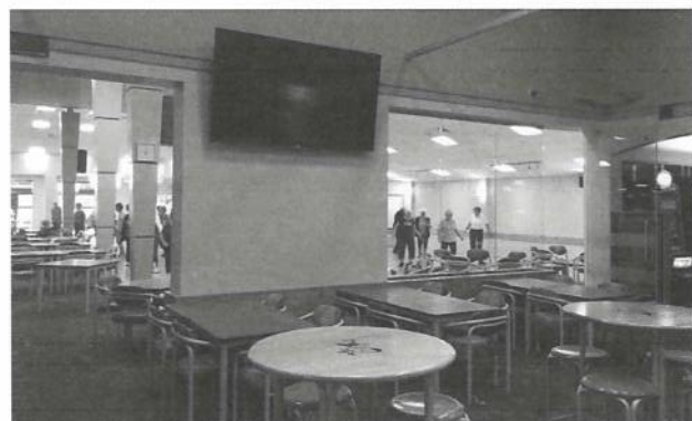
VIEW FROM BAR AREA SHOWING SOLID AREA OF THE WALL
